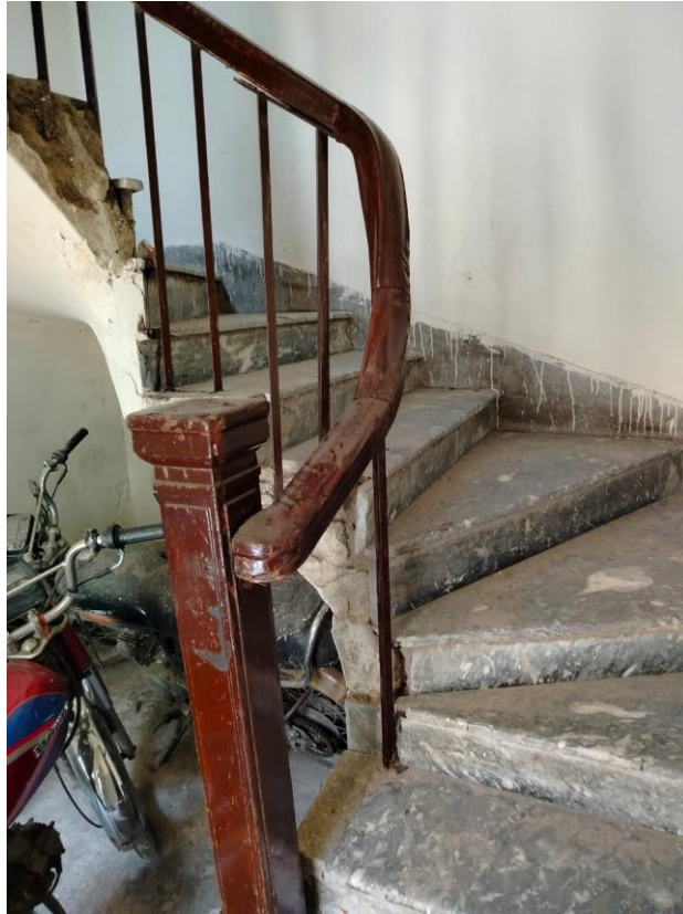
Plate 8 A: Staircase railing in its original form
