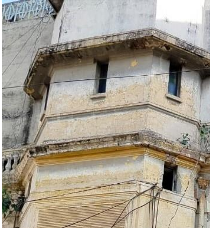
Plate 11 C: Small three directional ventilators
