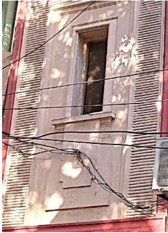
Plate 11 B: Stucco Decoration beneath the window
