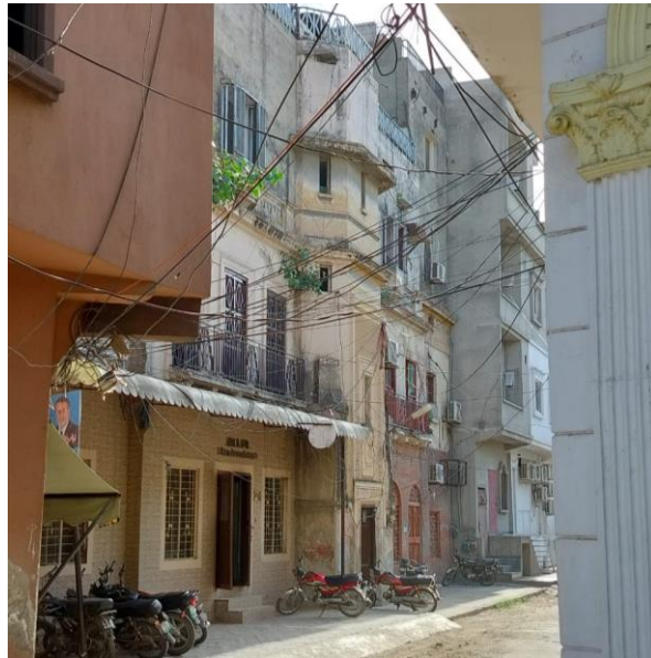
Plate 7: Northern side of Kapurthala House (second entrance doorway)
